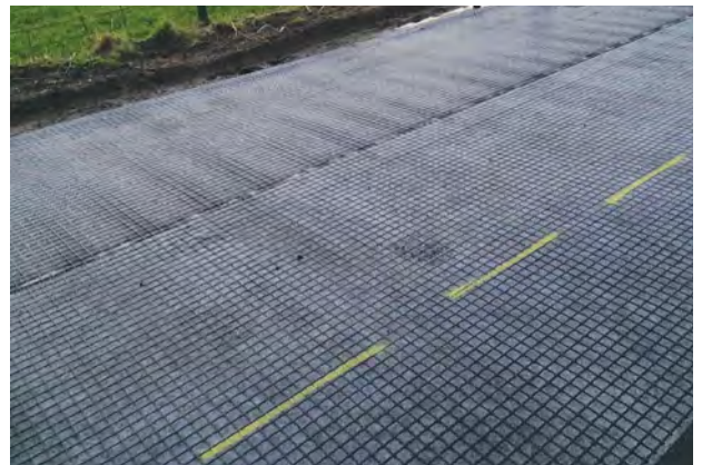
Tensar AR-GN can provide resistance to fatigue cracking and minimise fracturing due to long-term differential movements in the subgrade.
