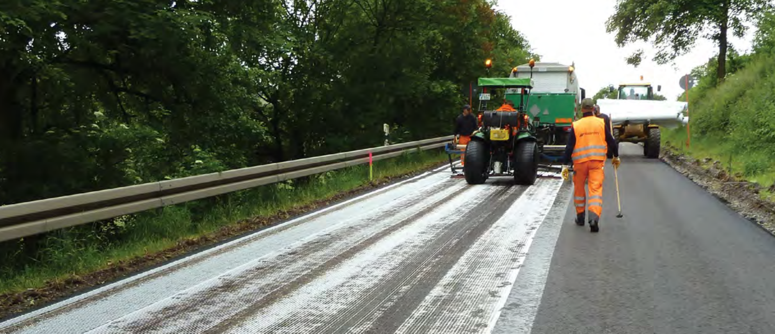
Installation of GlasstexGrid RN is straightforward.
