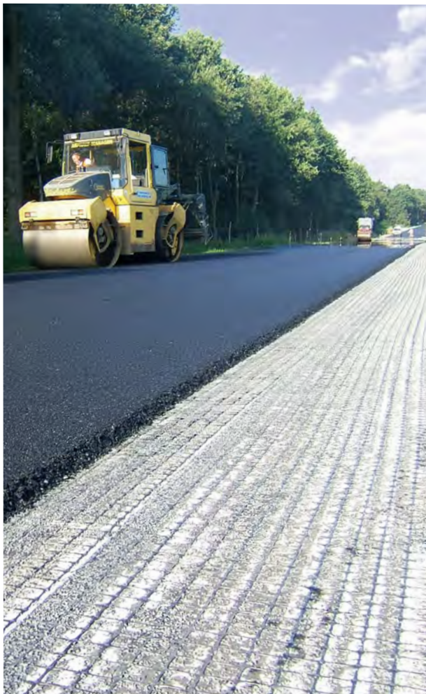
Tensar AR-GN bonds well on to the underlying surface to allow paving directly over the grid.
