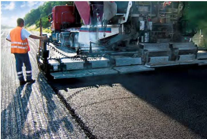
Paving takes place directly over the Tensar AR-GN
