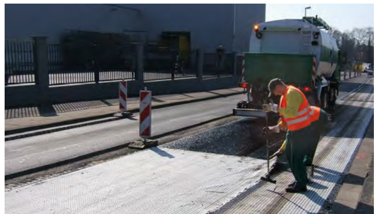
A simple overlap joint for Tensar Glasstex. Refer to installation guidelines for specific overlap instructions.
