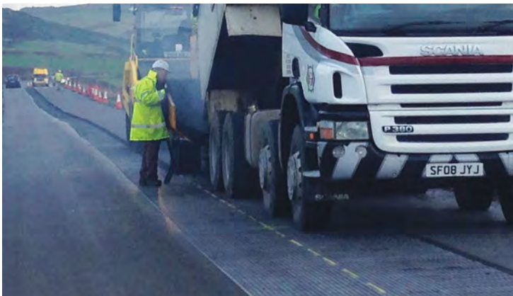
Tensar AR-GN can provide resistance to fatigue cracking and minimise fracturing due to long-term differential movements in the subgrade.
